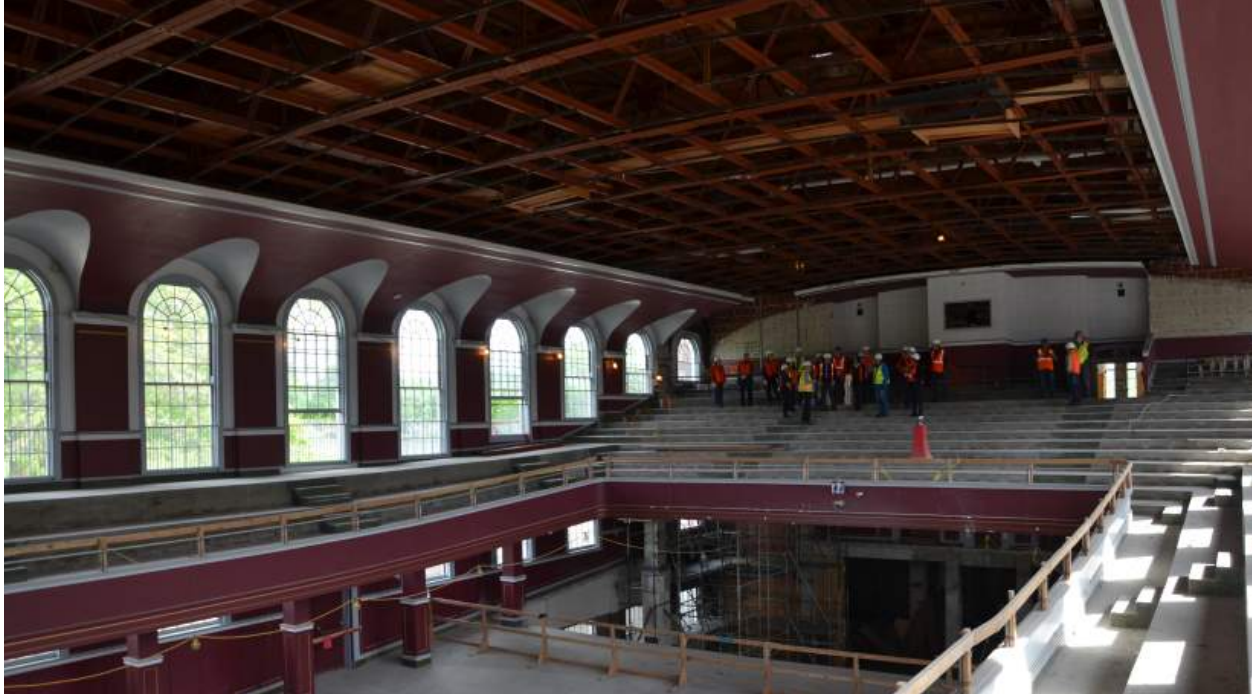
Franklin High School former auditorium under conversion to library
