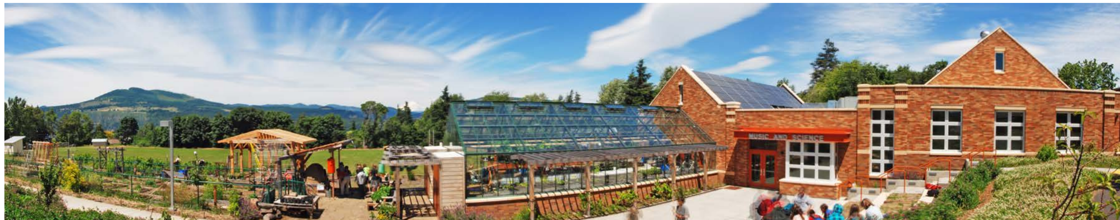
Hood River Middle School learning garden, green house and rooftop photovoltaic array
