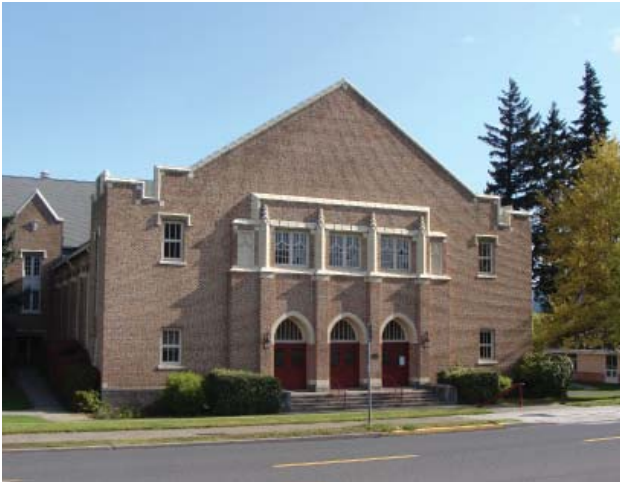
Existing 1927 National Historic Register Building
